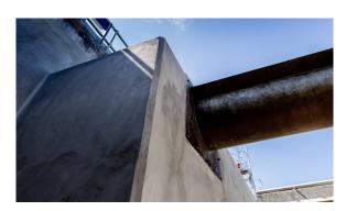
MasterSeal 586 – This was used for reinstating the damaged cover layer, applied in a thin coat it offers full protection of the underlying concrete and steel.
